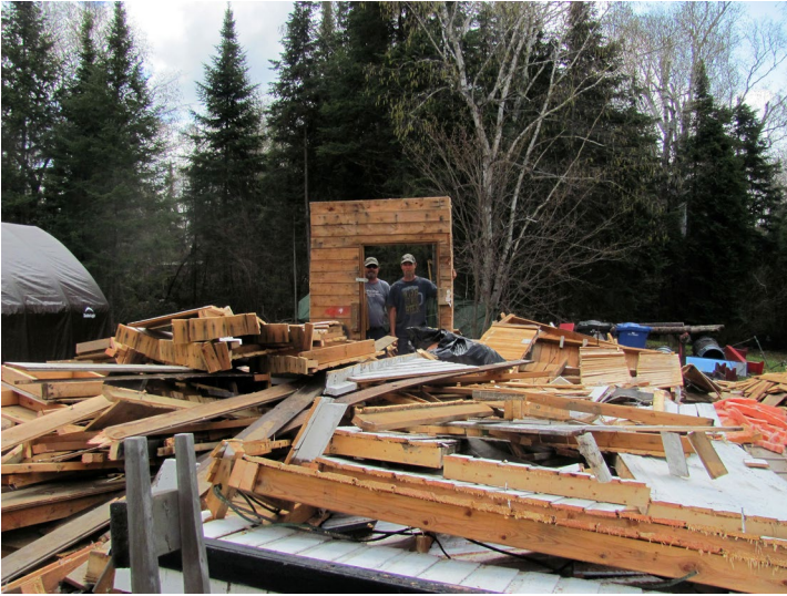
The demolition team of two
