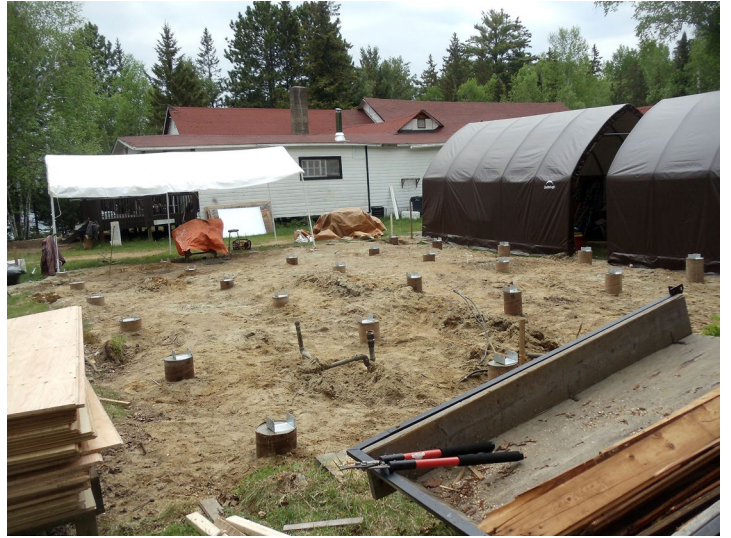
New foundation pillars
