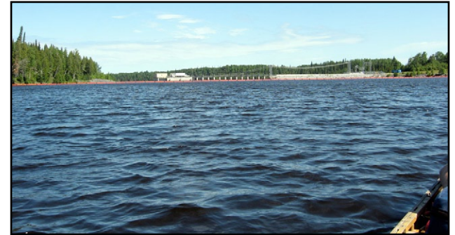
Approaching Smokey Falls Dam
